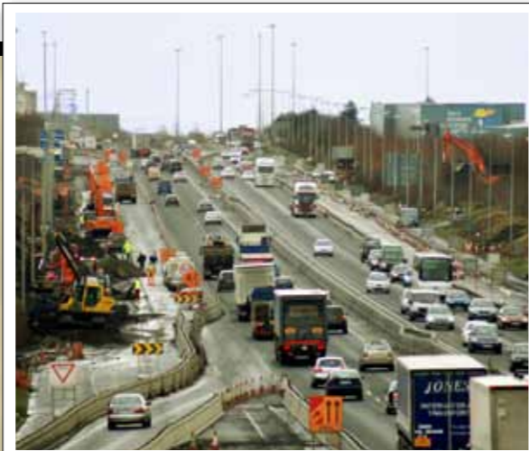
M50 Mainline Works
