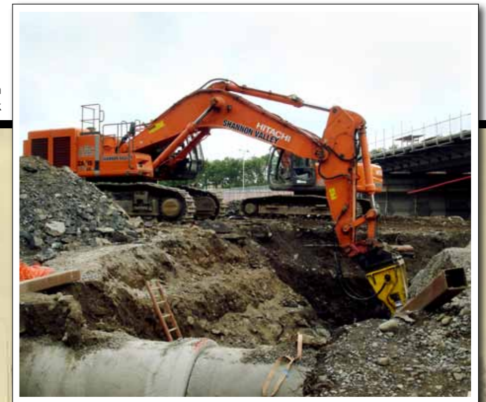
Drainage 7m deep in Rock
