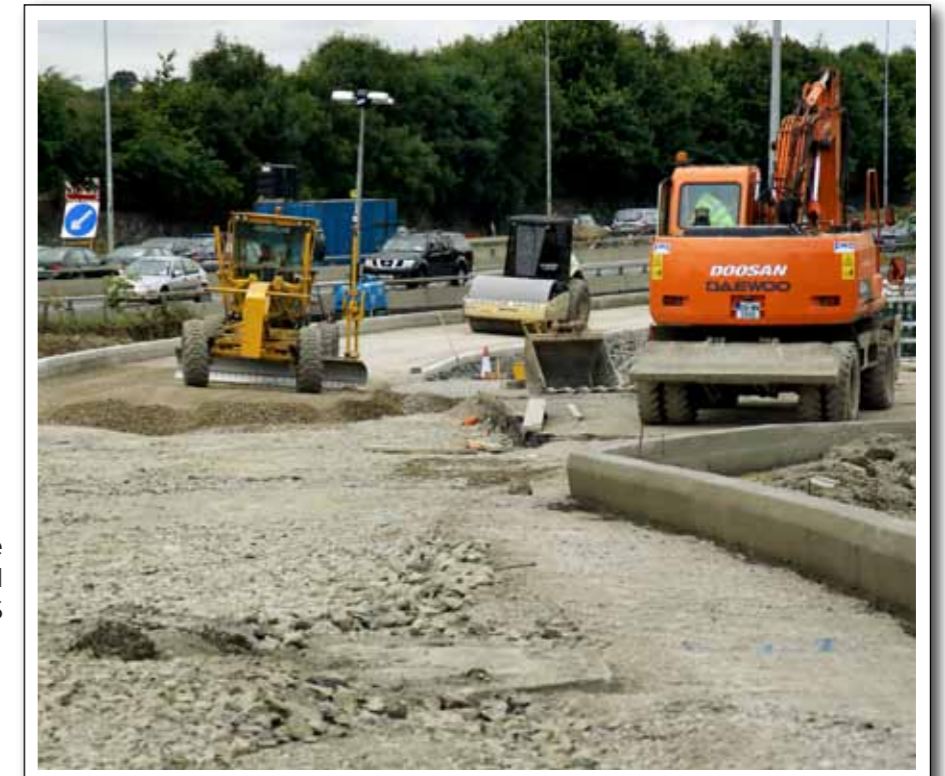
M50 Interchange works using road graders with ATS
