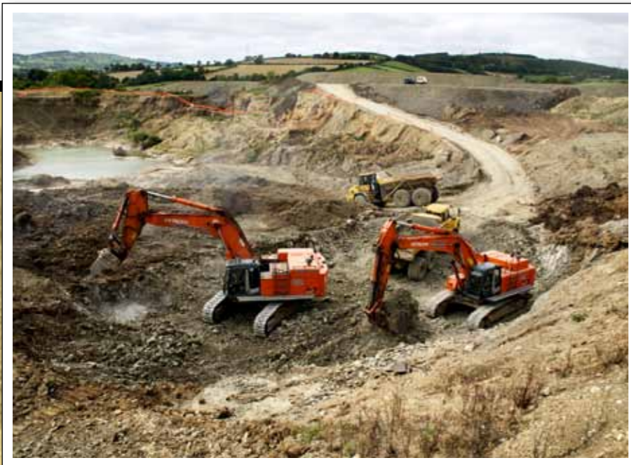
Rock extraction and haul road construction
